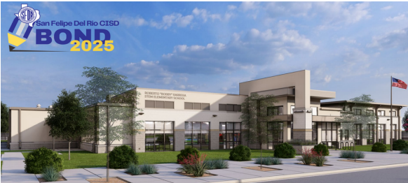
Roberto "Bobby" Barrera STEM Elementary School Project
